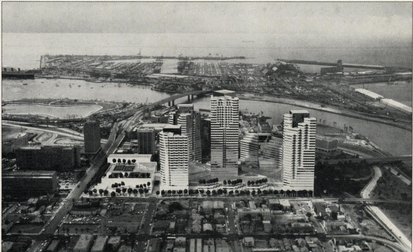
This summer will witness the ground breaking on the $550-million Greater Los Angeles World Trade Center at Long Beach. When completed in the early nineties, the center will sprout four office towers and a yet-to-be-awarded world-class hotel, but more important, its strategic position next to the burgeoning Los Angeles/Long Beach Port Complex promises to make the center the financial pivot point of Pacific Rim trade.
